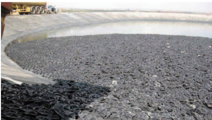
Hexa-Cover® Floating Cover BULK delivery and installation:
