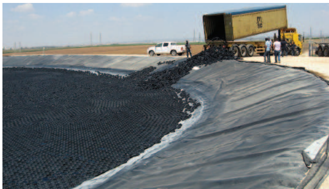
Hexa-Cover® Floating Cover BULK delivery and installation:
